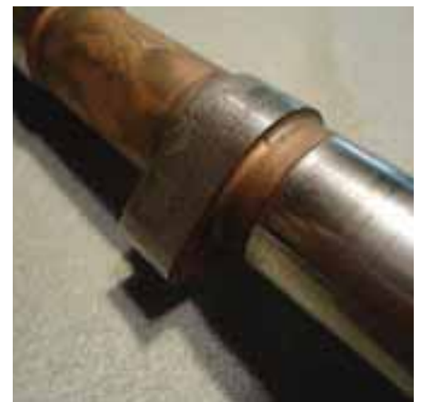
Corroded cam, typically through low use or poor maintenance.
