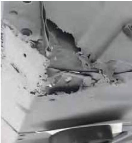
This is what showed up under prior 'repairs'...
