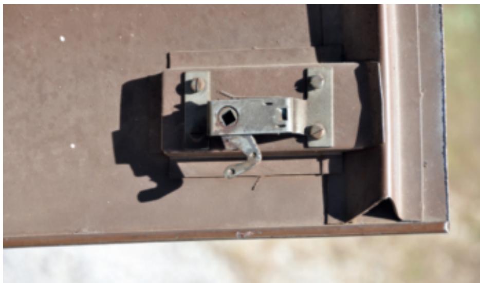
The inside of the outside latch. A version of the D-Type part.
