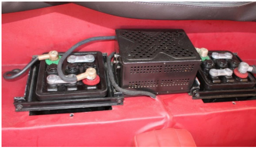
View of Batteries uncovered.
